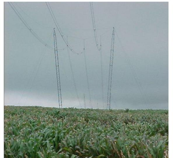
Figure 4: Photo of Cross Rope Suspension Tower
