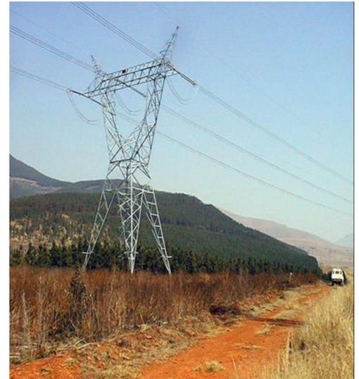
**Figure 6: Photo of Self-supporting Suspension Tower**
