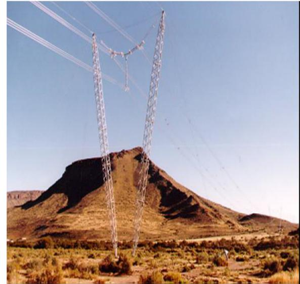
Figure 2: Photo of Guide V Tower
